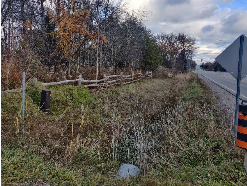
Image 7: Disturbed road right of way, no potential.
