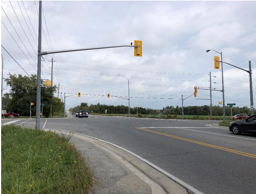
Plate 4: 20 th Sideroad, looking north to the intersection with 7 th Line in the central portion of the study area.
